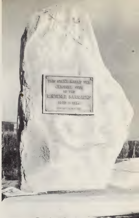
A stone marks the site of the first Mounted Police barracks at Fort Calgary. The site was marked near the present Canadian National Express depot in 1917.
